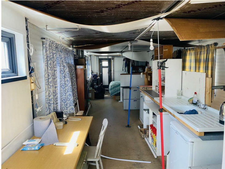
Double drainer sink unit, double glazed window, power point, doors to decking area.
